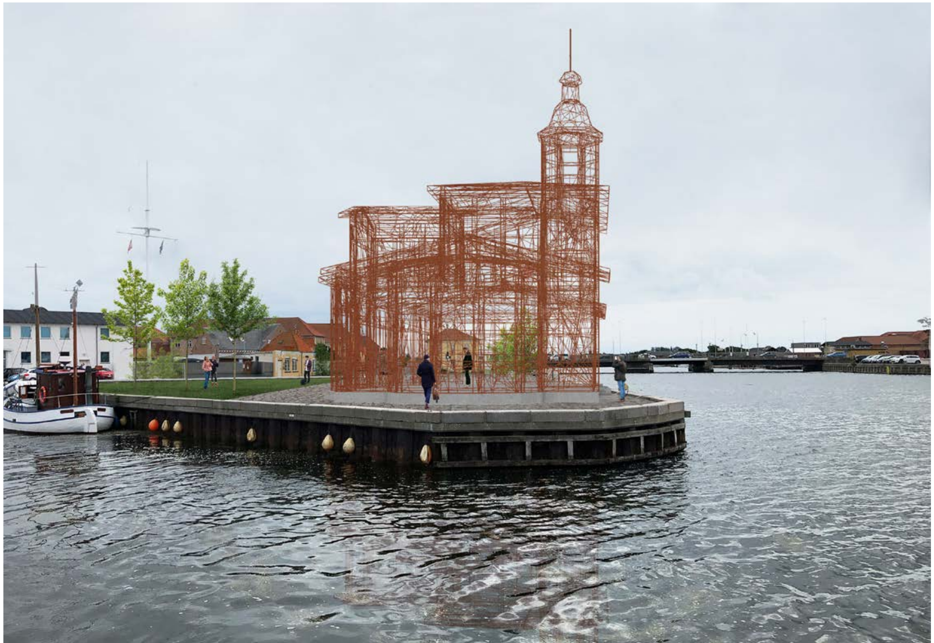
Optimised triangulated mesh, 38,5 tonnes, perspective view in a context
