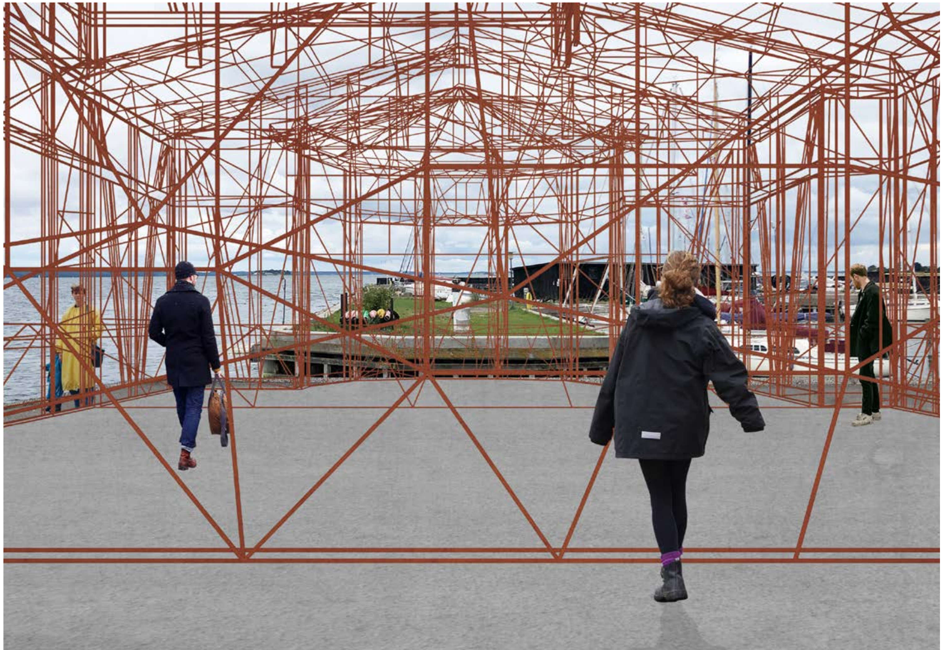
Optimised triangulated mesh, 38,5 tonnes, perspective interior view in a context
